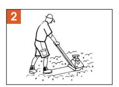
Lay road base and compact with a plate compactor. If the road base if very dry add a little water. If thicker that 100mm compact in layers. (55-75mm for a walkway, 150-200mm for a drive way), if laying on clay or fine sand use geo-fabric first.
