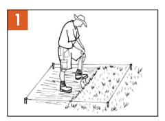
Prepare an area large than the paved area required. Clear area of all vegetation bark or soft soils. Check that finished height is not going to be higher that a door opening. Use
